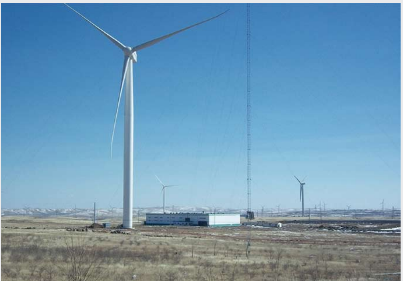
State Grid Project, China
